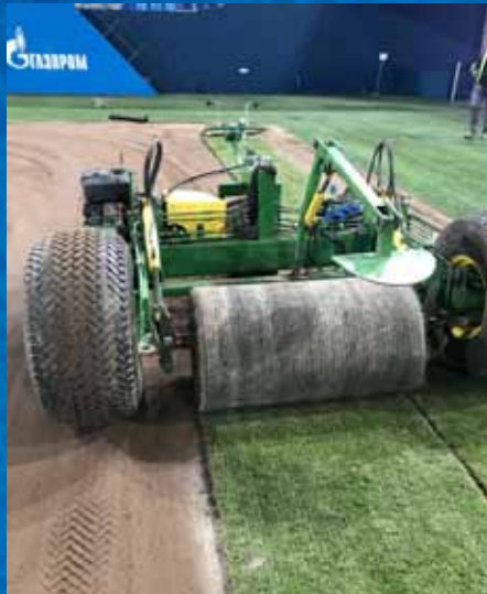
Turf installation
